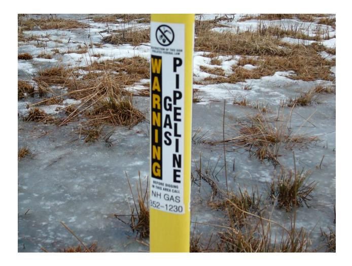
Once the gas arrives, New Hampshire Gas Corporation distributes it through underground pipelines safely and reliably to its customers. These pipelines underneath the street are vital to the utility infrastructure. Because many of these distribution lines are not marked, it is critical that people use the one call system prior to any excavation. When excavation work is planned, the pipelines are identified with yellow paint markings, stakes or flags.
