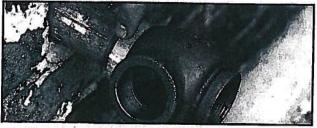
6 When the fitting is properly tightened, check that the yellow line on the nut and the yellow line on the body are together and positioned in the direction of the meter set. The yellow lines must meet.
