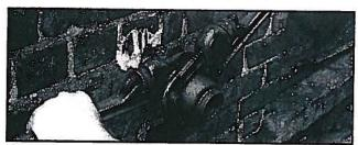
5 Tighten tee body until body and nut meet while holding the nut secure with locking wrench. The fitting cannot be over tightened because of the engineered mechanical stop.
