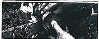
Stab plastic tubing into the POSI-LOCK® Basement Tee until it bottoms. You can hear it and feel it. Visually check by looking into open end of the tee.
